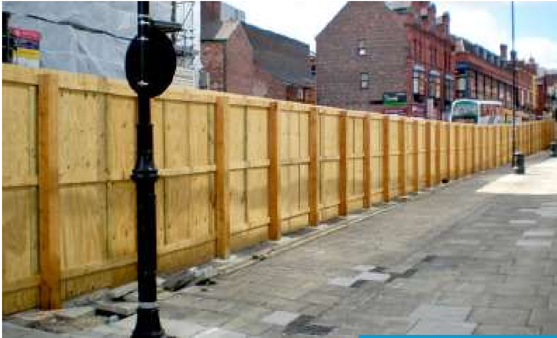
Fig 8, Post in hole hoarding
