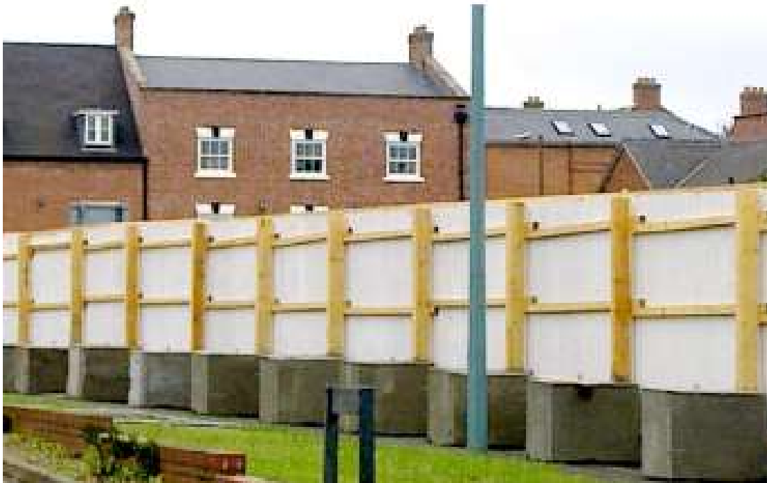
Fig 9, Kentledge Block hoarding.
