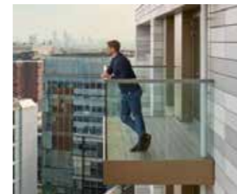
5 - Glass Balustrade to Balconies Generally; Square Top Railing and Edge to Selected RAL Colour
