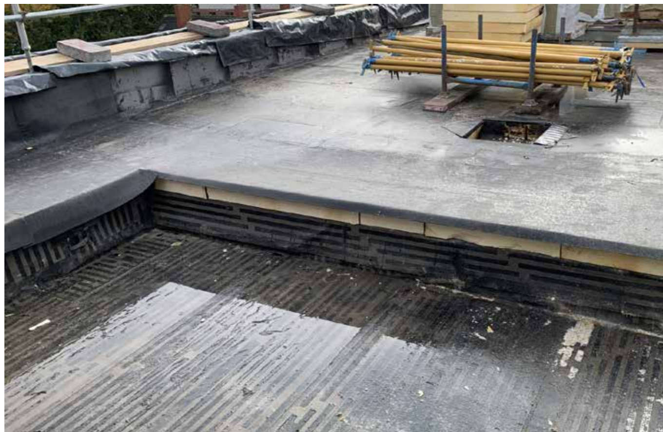
Recessed balcony picture showing step needed during the construction process
