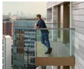
5 - Glass Balustrade to Balconies Generally; Square Top Railing and Edge to Selected RAL Colour Generally, Soffit to Match Brick Colour
